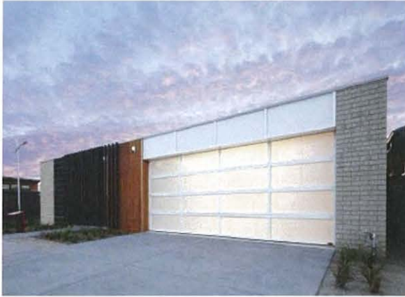
Figure 1 Garage presentation to the street
