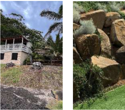
Tomaree Lodge, Building 01 and Vegetation.
