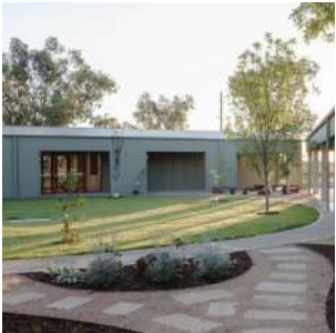
Project: Murrin Bridge Preschool + Community Centre / Supercontext
